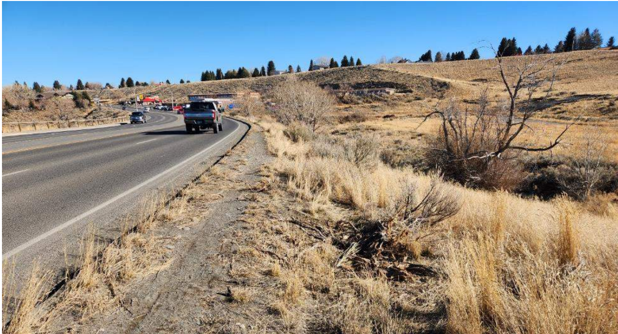
Figure 74. Area of Yellowstone Avenue with Sulphur Creek culvert
