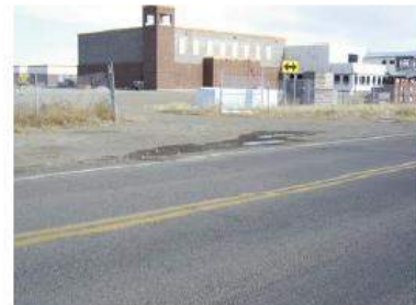
Sidewalks in Front of New Sunset Elementary School
