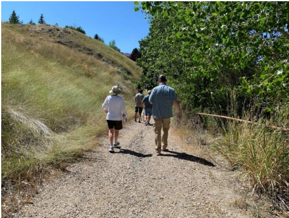
Figure 10. The walk audit followed the granular path down a slope which was experiencing erosion due to stormwater runoff. The eroded surface negates the path's ADA compliance in this area.
