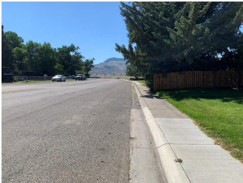
Figure 17. Throughout Cody, many sidewalks are placed at the back of the curb. This places people walking closer to motorized traffic than if a landscaped buffer were between the vehicular and pedestrian spaces.
