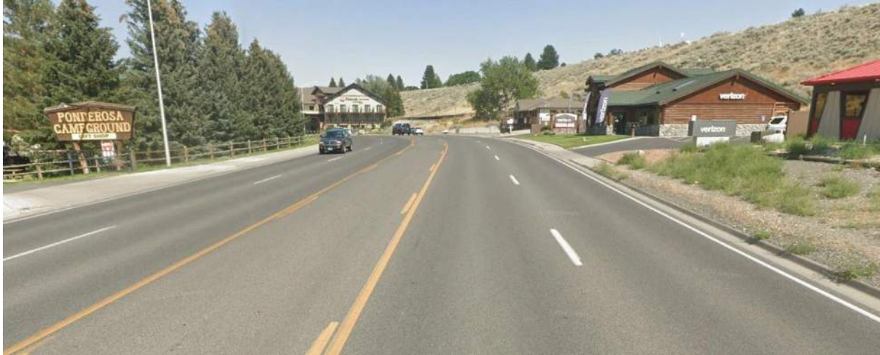
Figure 31. Section of Yellowstone Avenue past the curve known by some locally as “the gauntlet” due to narrow shoulders. Also note the missing sidewalk on the south side of the highway (right side of picture).
