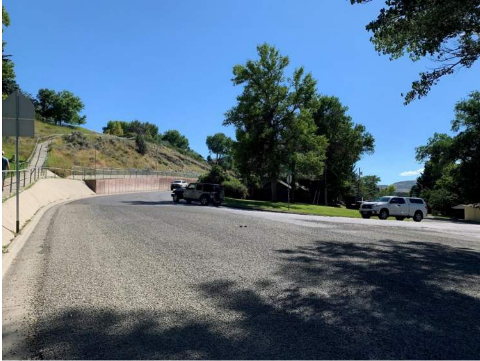
Figure 24. Motorists approaching from the stop sign at the right of the photo may have difficulty seeing oncoming traffic from the right (taken at the Canyon Avenue, 11th Street, and old South Fork Avenue intersection).
