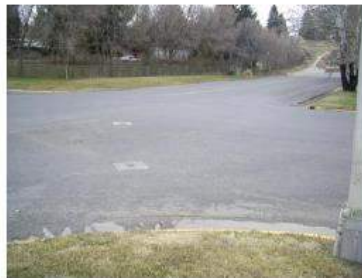
Additional Sidewalks Needed Along 11 th Street
