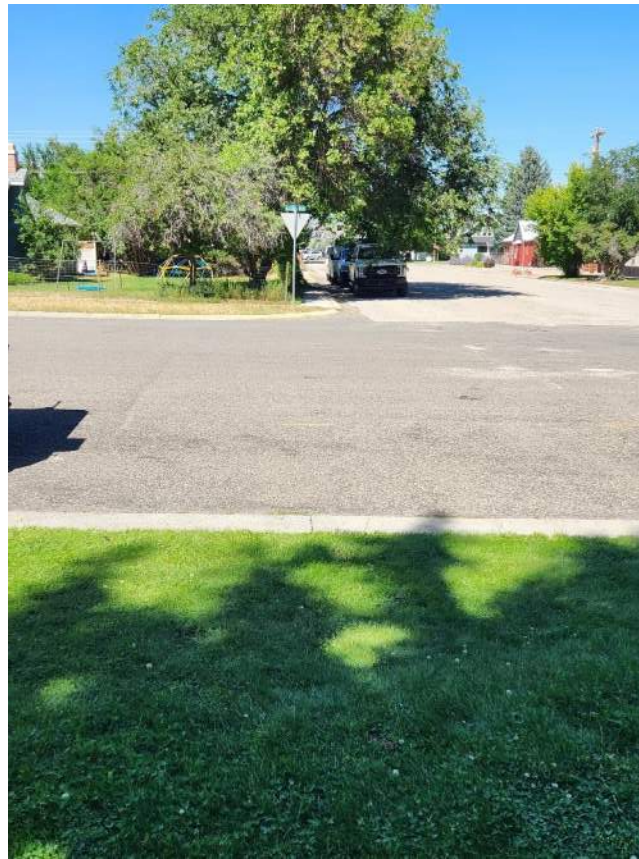
Figure 12. No ADA access from path (from photo above) across Alger Avenue to 15 th Street.
