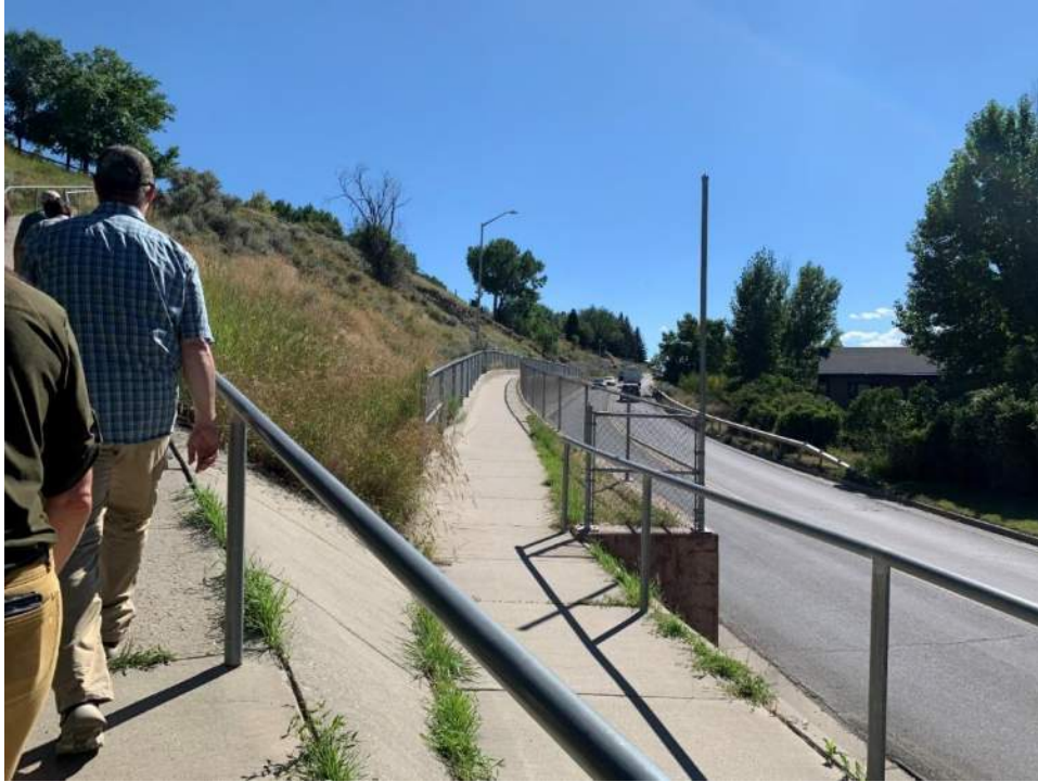
Figure 26. Fences and railings improve the sense of safety while walking along the sidewalk along 11 th Street which is placed at the top of a retaining wall.
